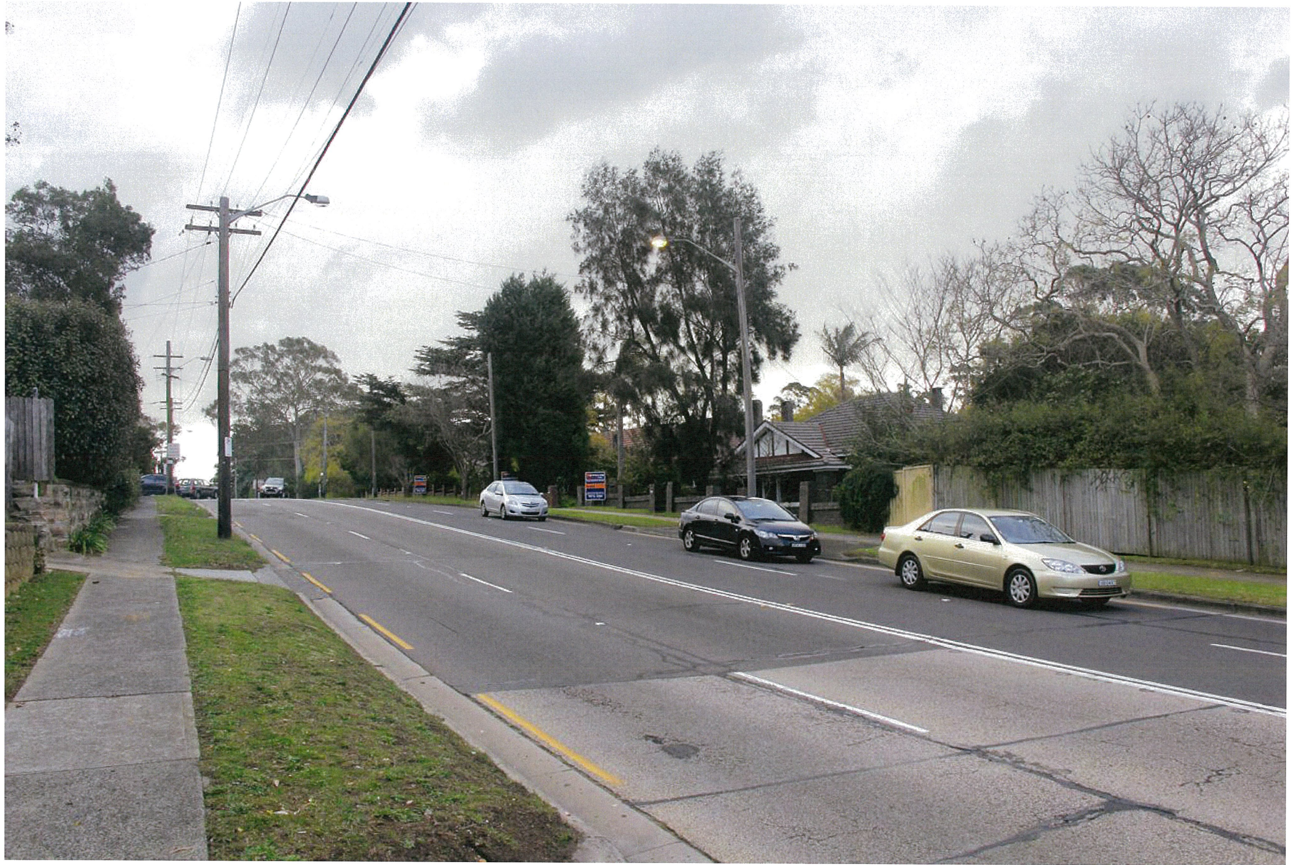
1 EXISTING VIEW AT EPPING RD
